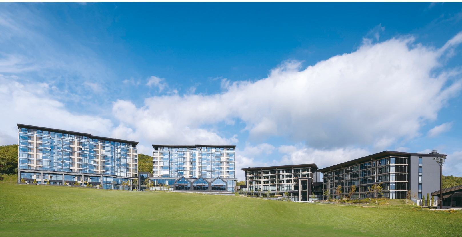
Park Hyatt Niseko Hanazono Residences and Park Hyatt Niseko Hanazono in Japan
